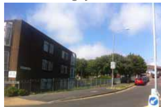
View from Whitehawk Road along Manor Way
